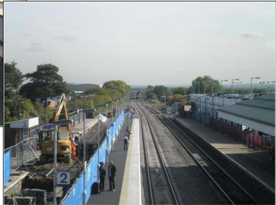
New layout – platform built out, and Up line has 100mph line speed
